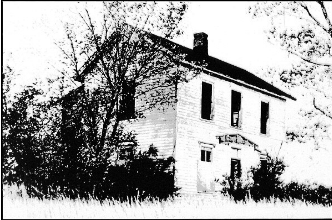
This house has been abandoned for decades but refuses to fall down
